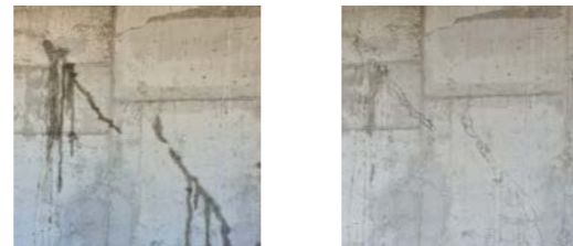
Below grade - Hospital, Denia, Spain
