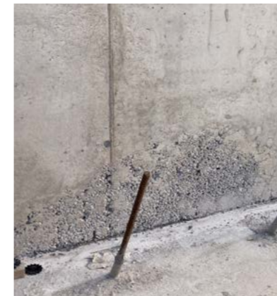
STRUCTURAL CONCRETE REPAIRS
