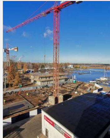
MARINE STRUCTURE POLAND
